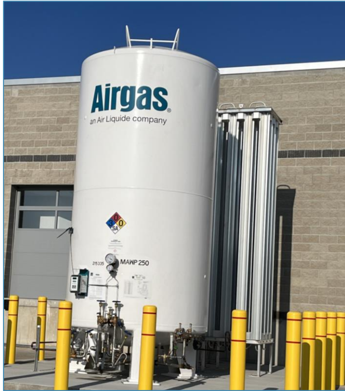
Nitrogen Tower for Uninterrupted N 2 Supply to Mass Spectrometers
